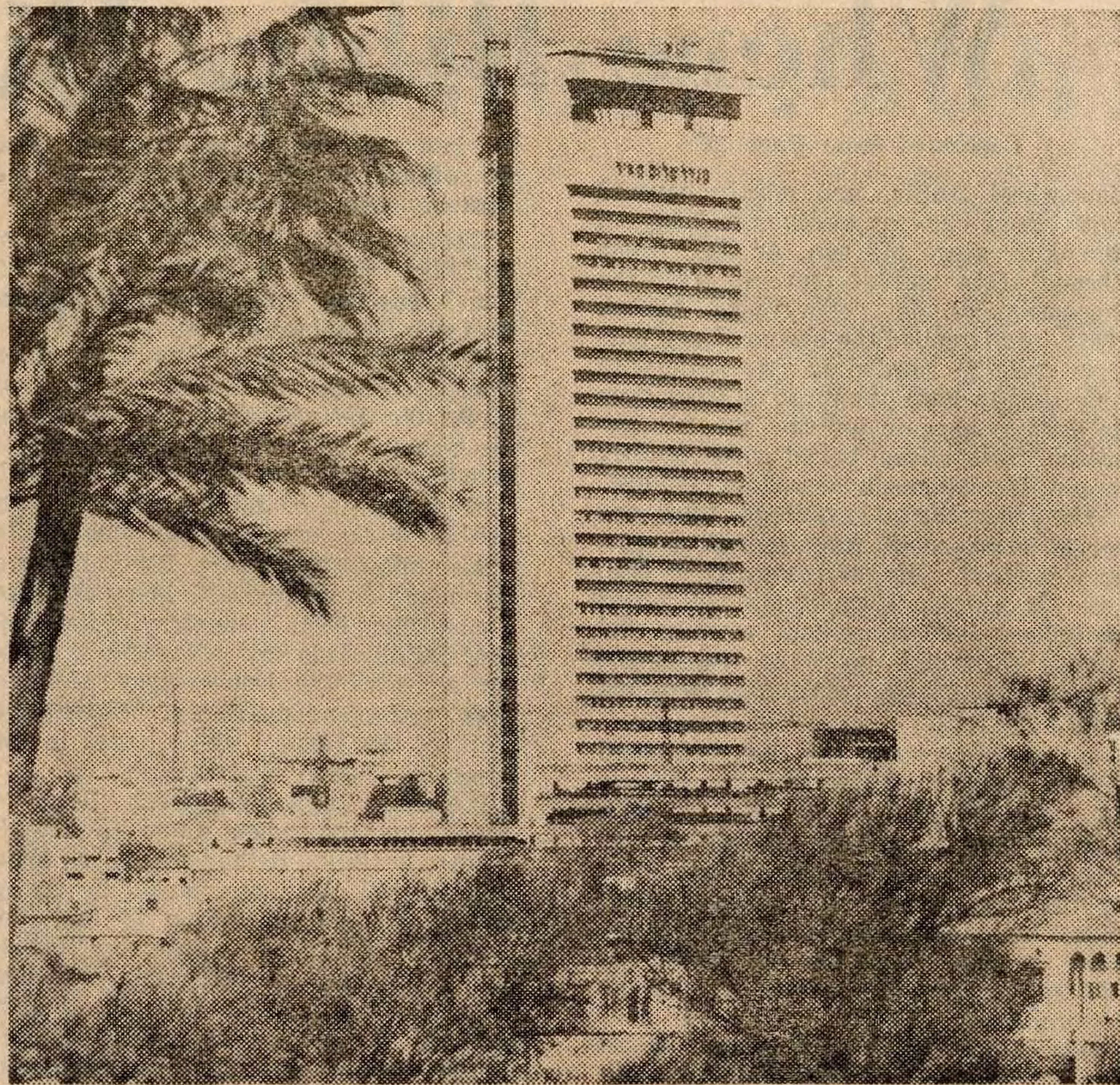
Shalom Tower in Tel Aviv, Israel's tallest building
