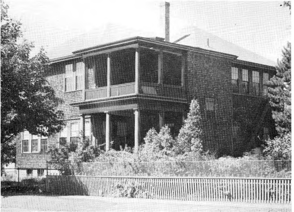
LISS MEMORIAL BUILDING
