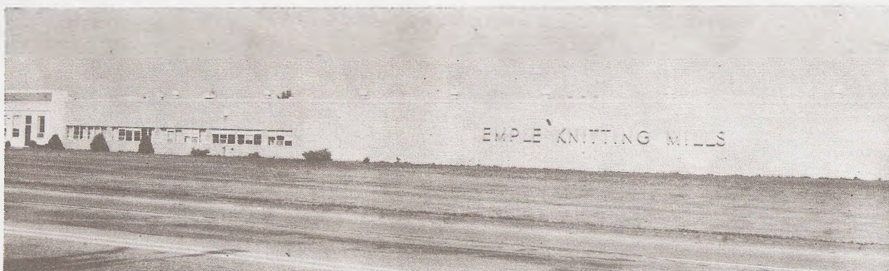
View of the 60,000 square feet Emple Knitting Mills plant on the outskirts of Brewer, Maine.
