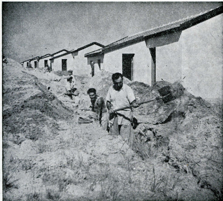
HOMES TO LIVE IN —Construction of 37,000 housing units in 1950 to speed the absorption of Israel's new immigrants is a major task to be met by American Jewry through the United Jewish Appeal. Here, modest homes typical of those being erected by the United Palestine Appeal agencies rise just outside Tel Aviv.
